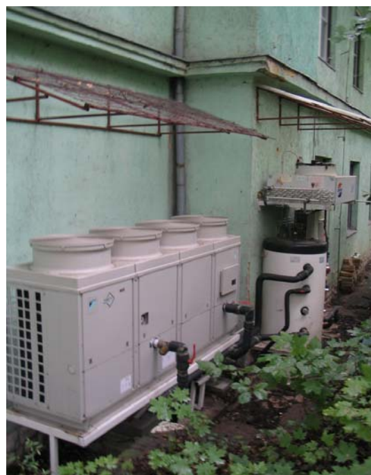
Water + air cooling system to support the SGI ICE
